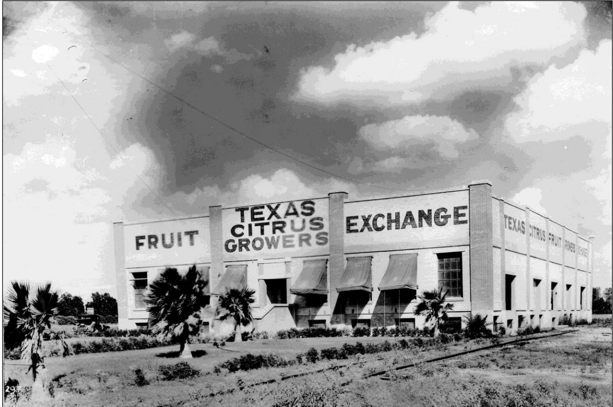
Exterior of Texas Citrus Fruit Growers Exchange, Sharyland, Hidalgo County, Texas, late 1920s, UTSA's Institute of Texan Cultures, No. 106-0196, Courtesy of Gayla Merrifield. Description: Photograph shows the brick building beside railroad track. Lower Rio Grande Valley, Texas-Mexico border.
