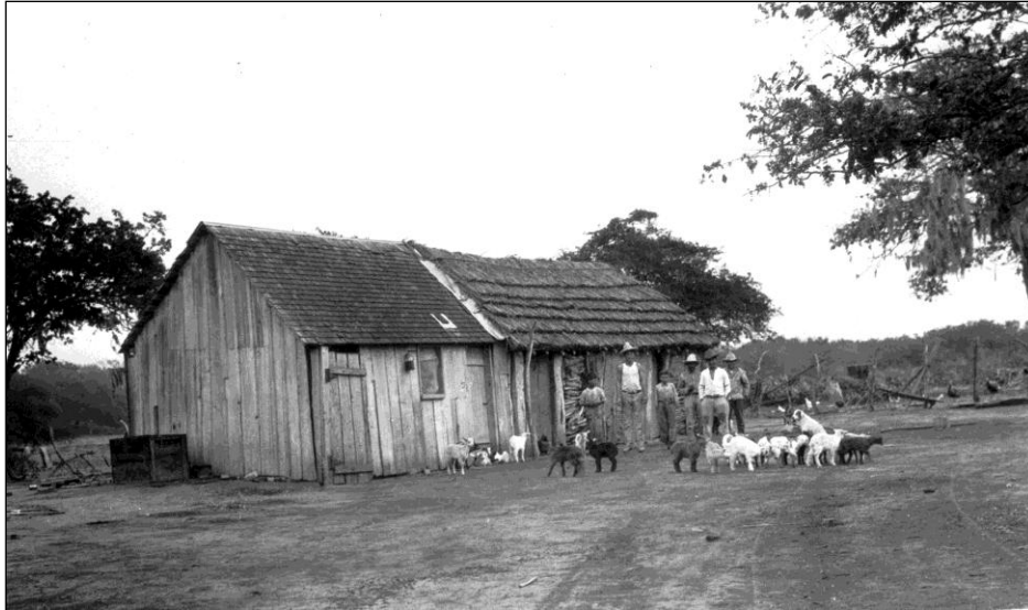
Group outside Rodriguez family home near San Benito, Texas, Between 1920-1930?, UTSA's Institute of Texan Cultures, No. 072-0889, Courtesy of Mrs. Clara Zepeda. Description: Photograph shows men and boys, surrounded by sheep, outside the house. Left portion of structure is board and batten; right side is jacal construction.
