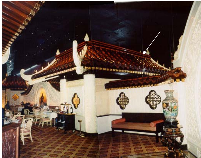
Figure 33. Mirrors above building façade create illusion of continuing night sky and complete building. Arrow shows the mirrors seam and where the roof ends at the wall.
