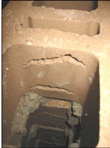
Figure 3.4: Cracked bricks
