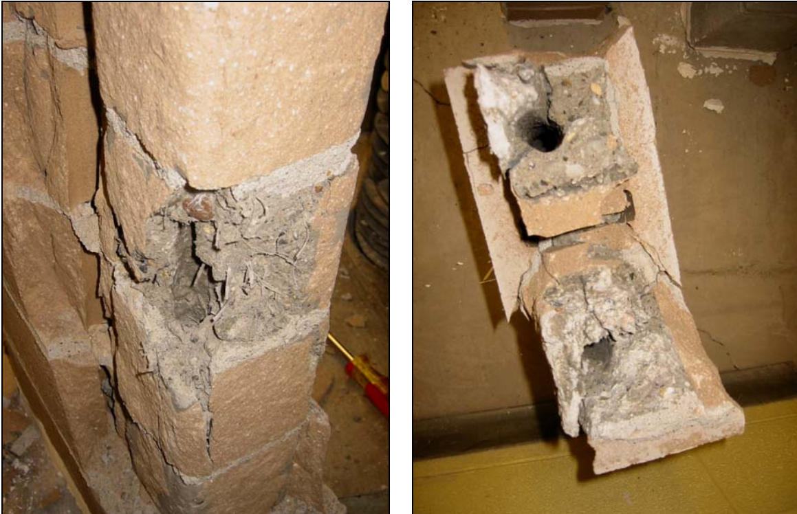
Figure 3.15: Holes in the grout due to the vibrator
