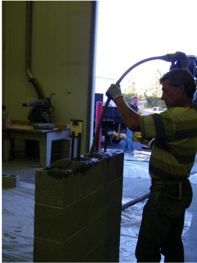
Figure 3.6. Grouting and Vibrating
