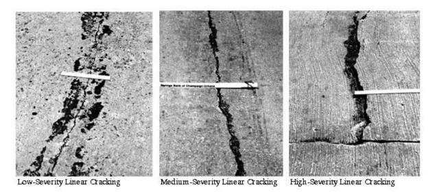
Figure 4.1: Severity of Linear Cracking (ASTM D6433, 2007 Figures X2.22-X2.24)
