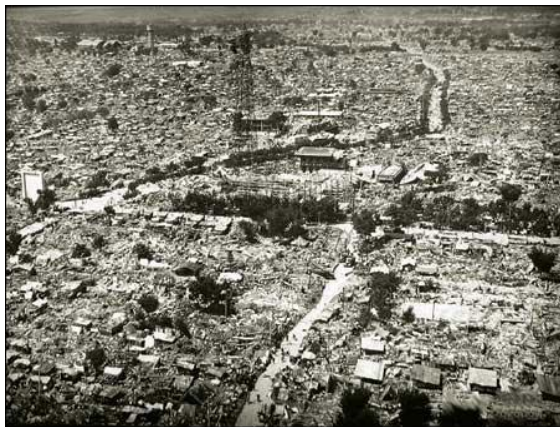
Figure 37. Ruins after Tangshan quake.
