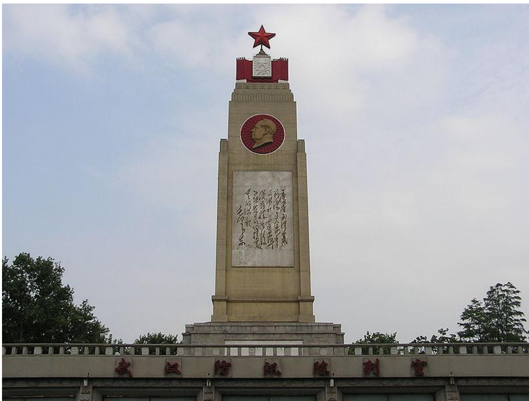
Figure 59. Wuhan 1954 Flood Memorial.
