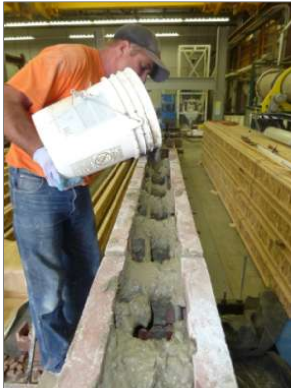
Figure 3.7: Construction Phase 2: Grouting
