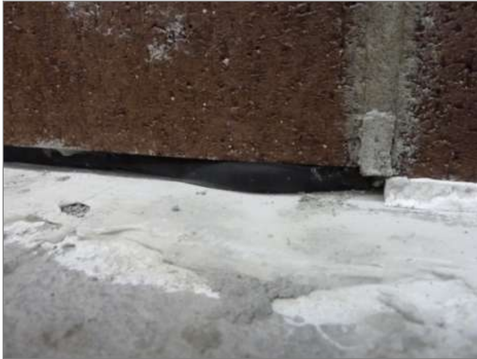
Figure 5.4: Lateral Expansion of Neoprene
