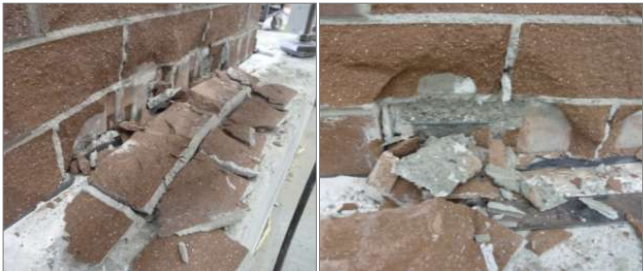
Figure 4.14: Spalling on East (left) and West (right)
