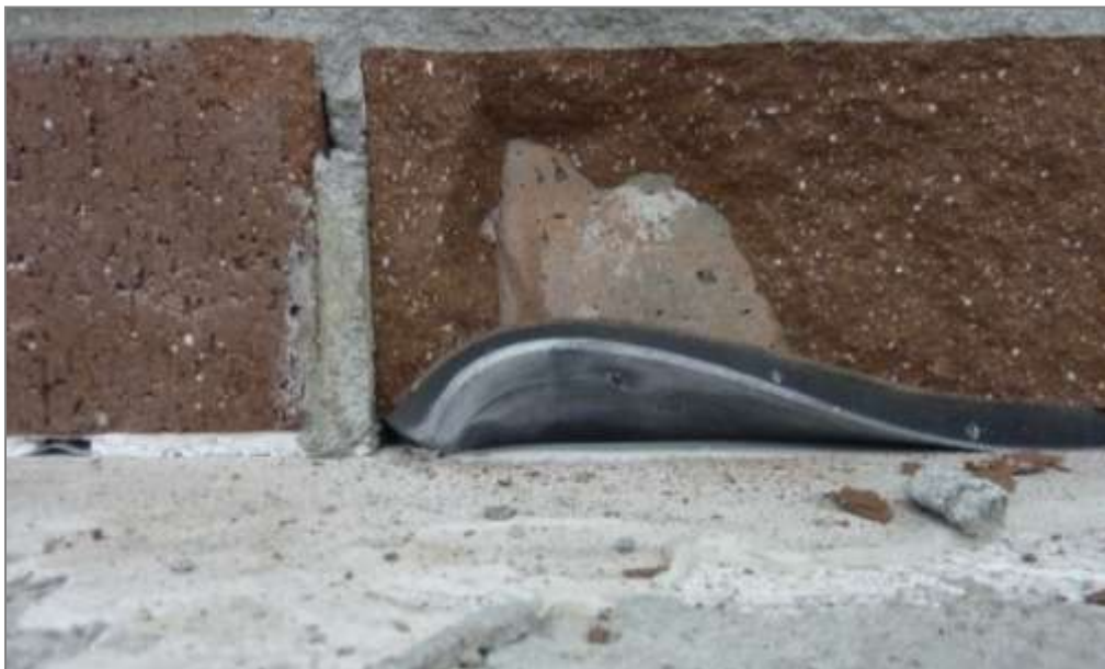
Figure 5.5: Neoprene Deformation in Panel 1
