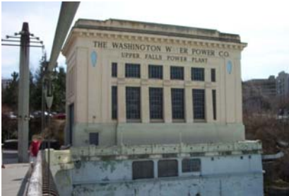
Fig. 25 Upper Falls Power Plant.
