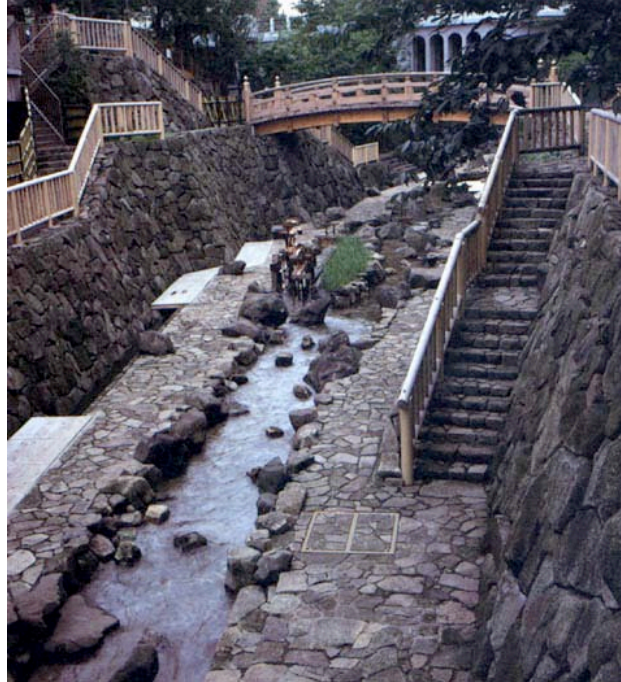
Figure 2-8. Basalt paving with a natural appearance, Tokyo, Japan. (from Elements and Total Concept , 1990)
