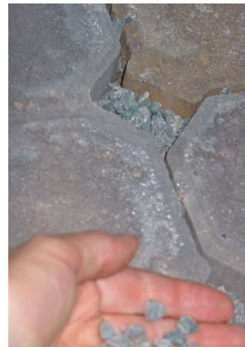
Figure 2.2-25. Aggregate-filled pavers in a residential driveway in Minneapolis, MN (Source http://www.marcy-holmes.org/projects/rainwater/5.html )
