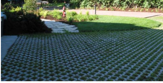
Figure 2.2-26. Pervious pavers using grass and soil media in paver pore spaces. (Left: http://revelle.net/LAKESIDE/photos/july/July-Pages/Image6.html , ; Right: http://er1.org/docs/sample_solutions/products/Landscaping with load-bearing grass paver systems.jpg )
