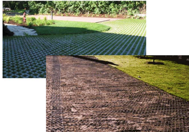
Figure 5.4-3. Grass pavers and mesh reinforced turf for swale edge reinforcement. Rubber/plastic plow blades may be needed to prevent tearing mesh reinforcement. See Ferguson (2005) for additional turf reinforcement methods (Source: Top - http://revelle.net/LAKESIDE/photos/july/July-Pages/Image6.html ; Bottom - http://grasstrac.com/case_univ_ga.htm )
