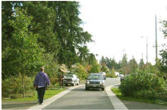
Figure 5.4-2. Narrow street with low/no curbs. Street edge swales can be used for plowed snow storage. Unlike this example, woody plant species should be placed away from roadside swale edges to avoid damage from plow blades. (Source: http://www2.cityofseattle.net/til/tours/seastreet/slide6.htm )
