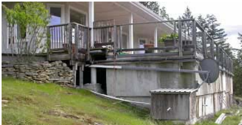
Figure 5.5-1. Cistern as deck foundation (Source: http://www.rainwaterconnection.com/rainwater_harvesting/basic_components.htm ).
