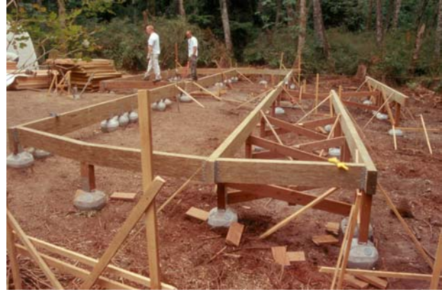
Figure 2.2-13. Diamond Pier™ minimal excavation foundation system used on Bainbridge Island, WA (Sources: Pin Foundations, Inc., Hinman, 2005, p. 129)
