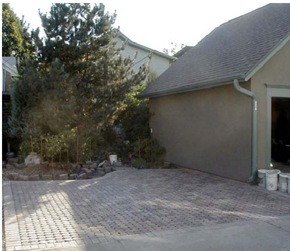
Figure 2.2-25. Aggregate-filled pavers in a residential driveway in Minneapolis, MN (Source http://www.marcy-holmes.org/projects/rainwater/5.html )
