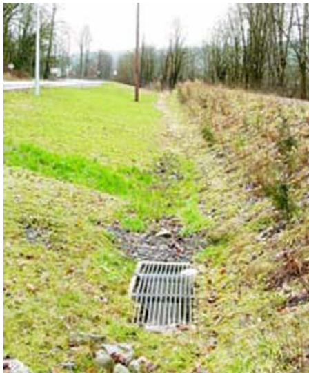
Figure 2.2-14. A biofiltration channel with outflow inlet (Source: http://www.wsdot.wa.gov/Environment/WaterQuality/Research/LinksLiterature.htm )
