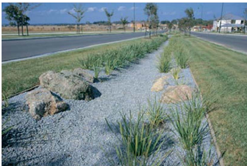
Figure 2.2-22. Infiltration trench with aesthetic elements, Melbourne, Australia (Source: http://wsud.melbournewater.com.au/content/treatment_measures/infiltration_trenches/overview.asp )
