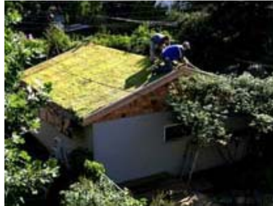
Figure 2.2-28. Left: mature vegetated roof. Right: installation of a commercially available vegetated-mat system. (Sources: Left, Liptan and Murase, 2000, p. 20; Right, http://marcy-holmes.org/projects/rainwater/6.html )
