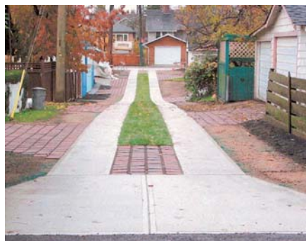
Figure 2.2-10. Reduce impervious areas in driveways and alleys by paving only the wheel tracks (Photo courtesy of Curtis Hinman)
