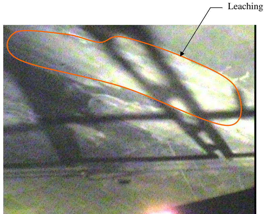
Figure 4.18 – Photo of Heating Location # 1 showing extensive discoloration due to leaching
