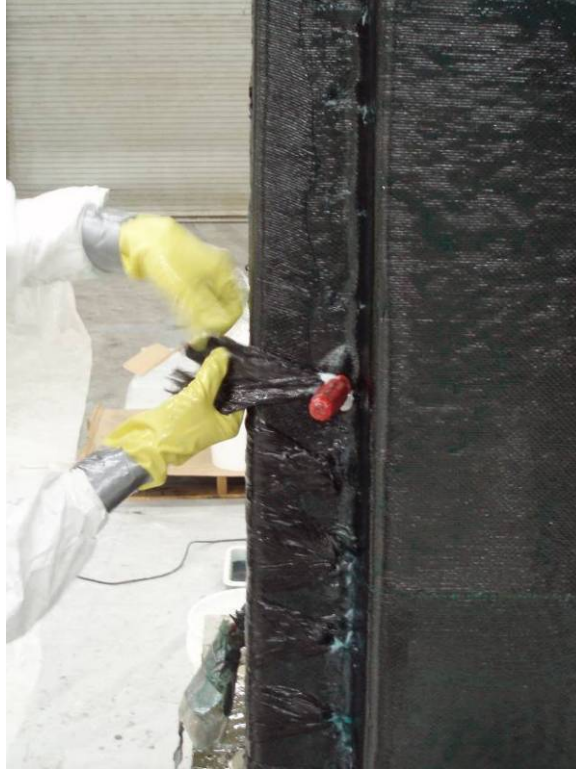
Figure 4.4.6 – FRP Anchor Installation
