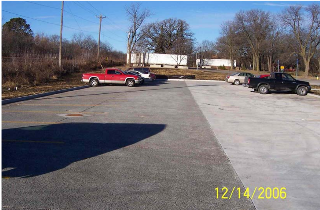
FIGURE 2.2: Finished parking lot, pervious on the left and traditional concrete system on the right (picture courtesy John Kevern)
