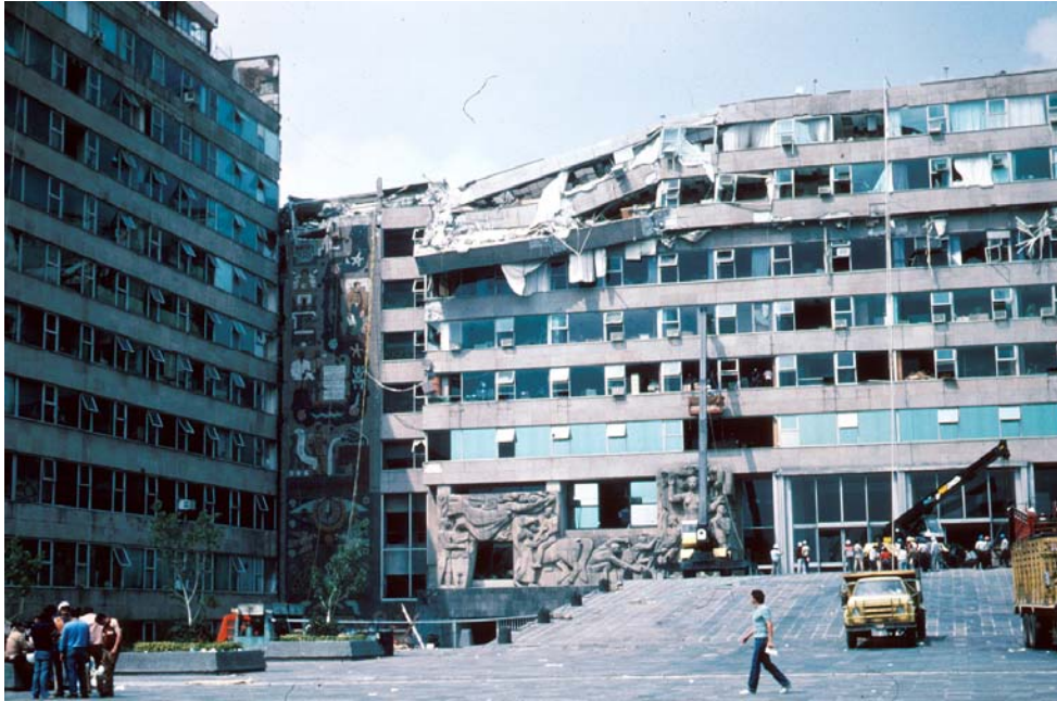
Figure 1.4 Damage to Reentrant corner and Upper stories of the Ministry of Telecommunications Building in Mexico City after the 1985 earthquake.
