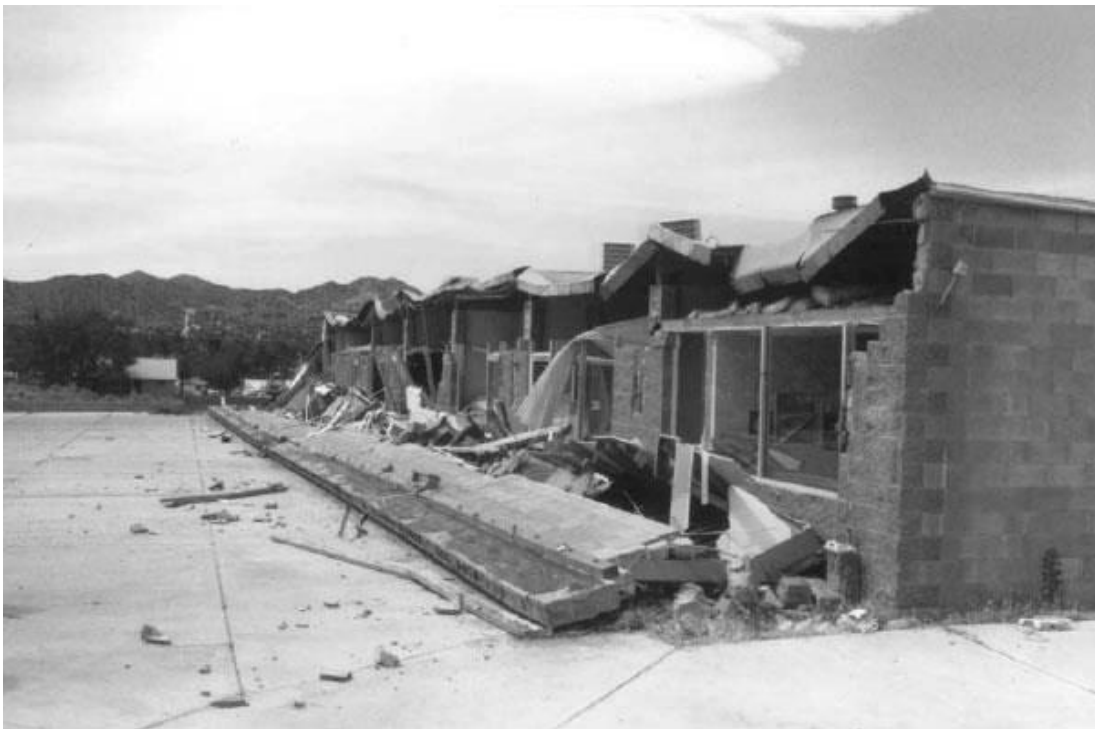
Figure 1.3 Out-of-Plane Wall Failure Example
