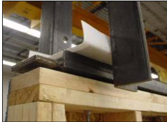
Lateral Bracing—North End
