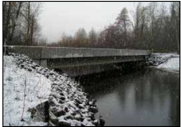
Figure 2: Skobob Creek (crossing SR 106), 1.83 m wide concrete box culvert replaced with a 37 m wide single span bridge (Barber et al., 2006)
