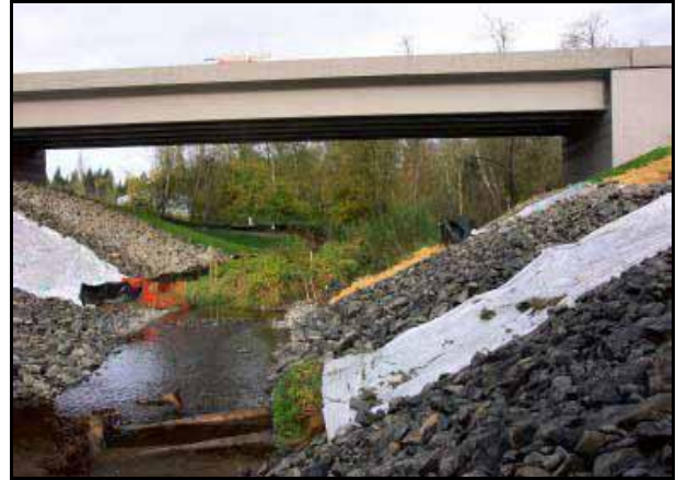
Figure 3: Taylor Creek (crossing SR 18), 1.52 m wide concrete round culvert replaced with a full span bridge for $2.14 million (Barber et al., 2006)
