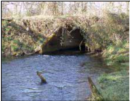
Figure 2: Skobob Creek (crossing SR 106), 1.83 m wide concrete box culvert replaced with a 37 m wide single span bridge (Barber et al., 2006)
