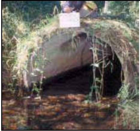
Figure 3: Taylor Creek (crossing SR 18), 1.52 m wide concrete round culvert replaced with a full span bridge for $2.14 million (Barber et al., 2006)
