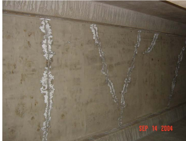
Fig. 1.3 Transverse, Full-depth Cracks Developed within 48-hour of Pouring
