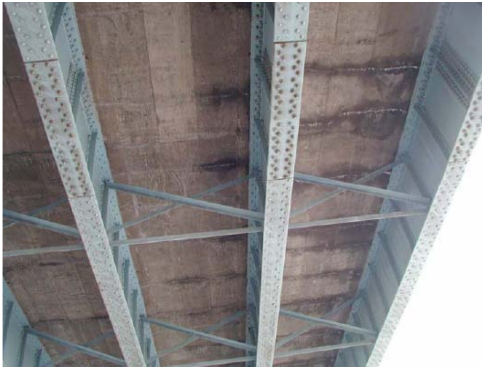
Fig. 1.2 Early-age Shrinkage Cracking in Concrete Bridge Decks (Crowl and Sutak 2002)
