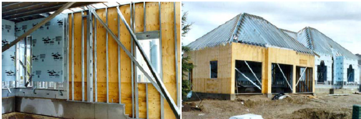
Figure 1-Typical Residential Construction Using CFS Framing with WSP sheathing (left: interior view of CFS wall; right: exterior view) (Branston, 2004)
