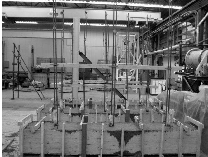
Figure A-3: Freshly poured foundations
