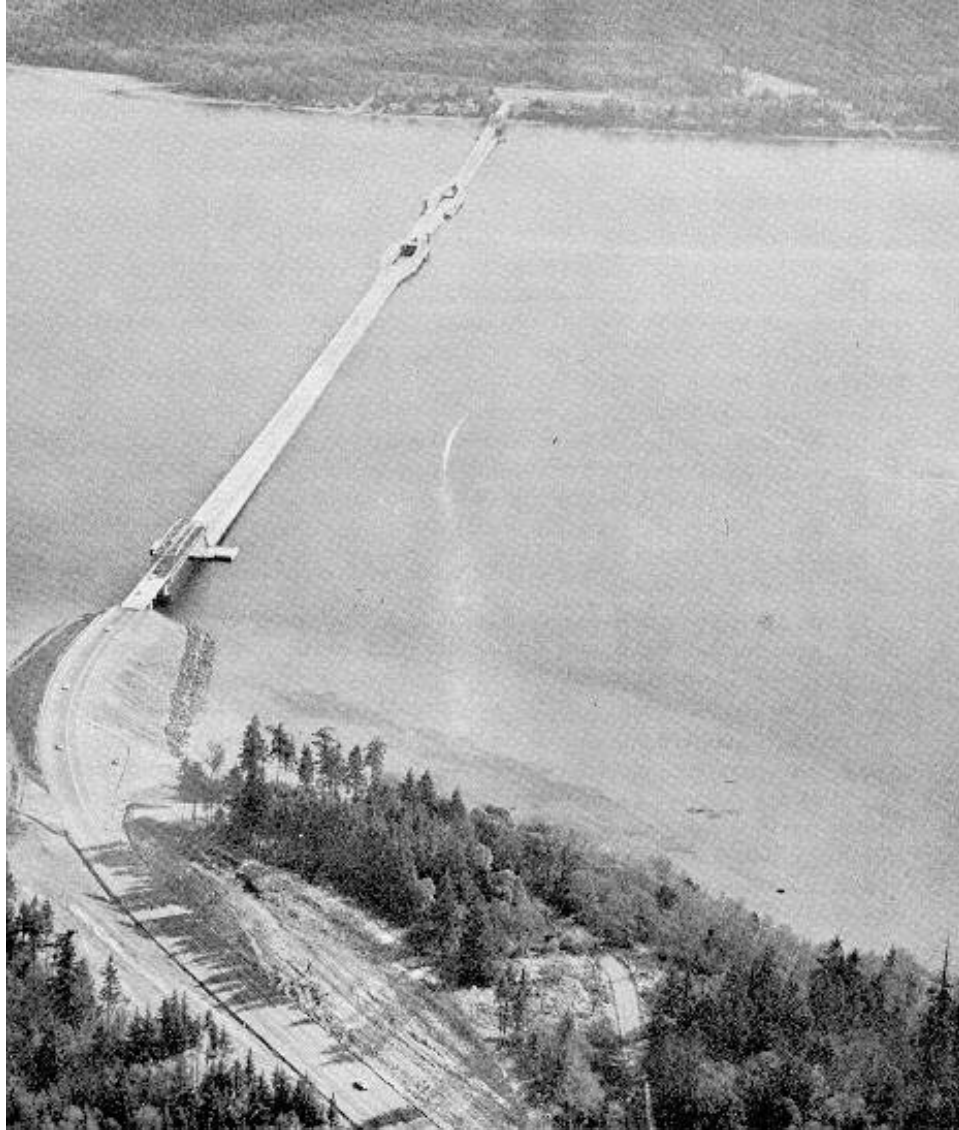
Figure 1.10 – Hood Canal Bridge Photo obtained from WSDOT Biennial Reports Image Library
