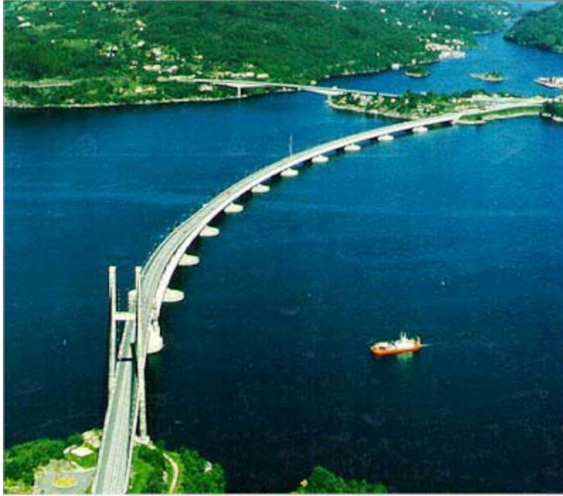
Figure 1.5 – Salhus Bridge Near Bergen, Norway
