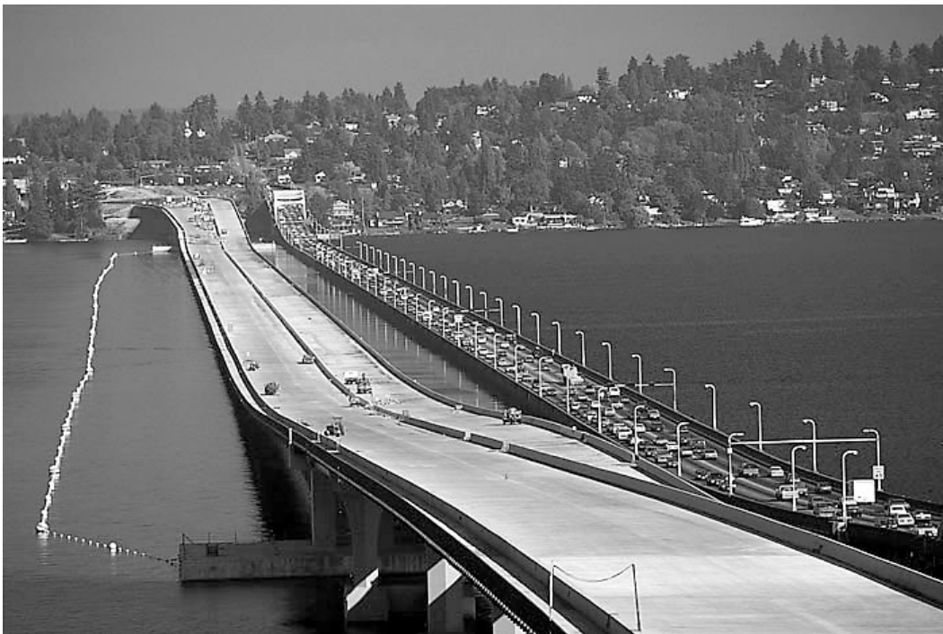
Figure 1.14 – HMHMB (Under Construction) & Original LVMB
