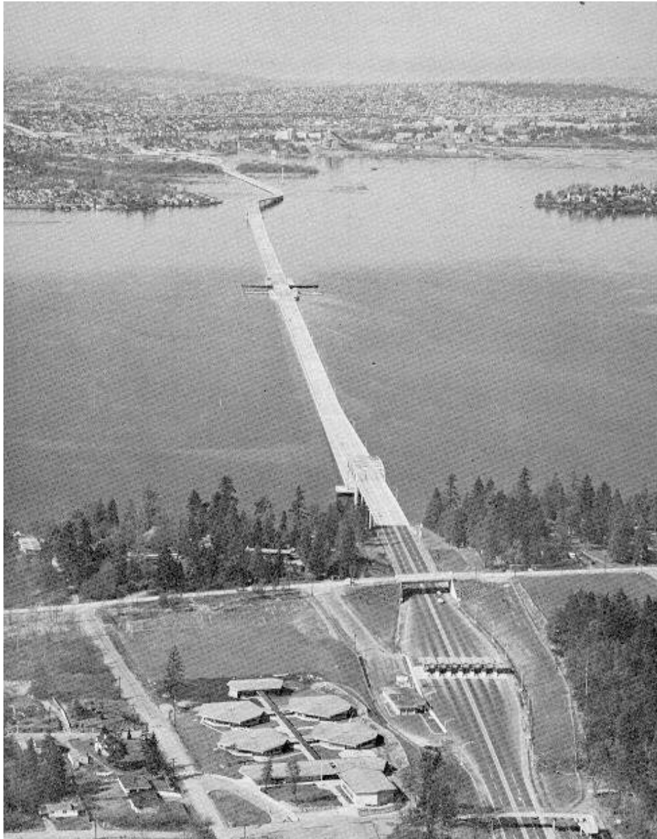
Figure 1.11 – Evergreen Point Floating Bridge, Looking West Toward Seattle Photo obtained from WSDOT Biennial Reports Image Library
