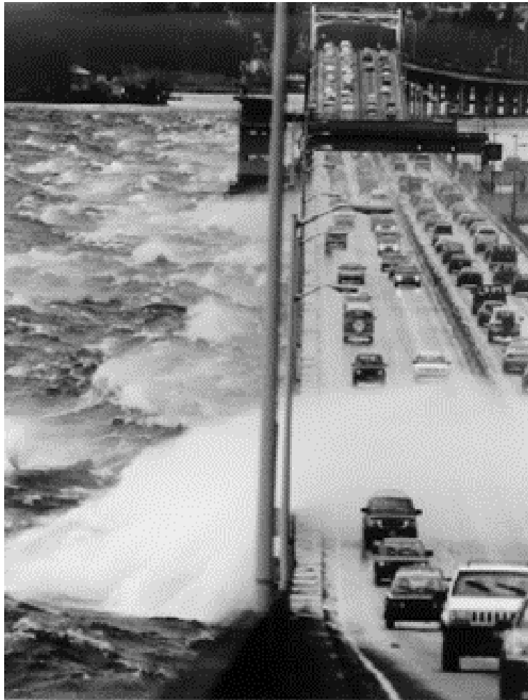
Figure 1.19 – EPFB Under Storm Conditions Figure obtained from: http://www.acec.org/EEA/pressrelease/520bridge.doc
