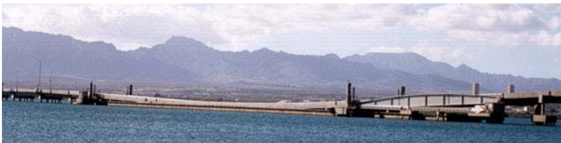
Figure 1.6 – Floating Drawspan of the Admiral Clarey Bridge, Hawaii
