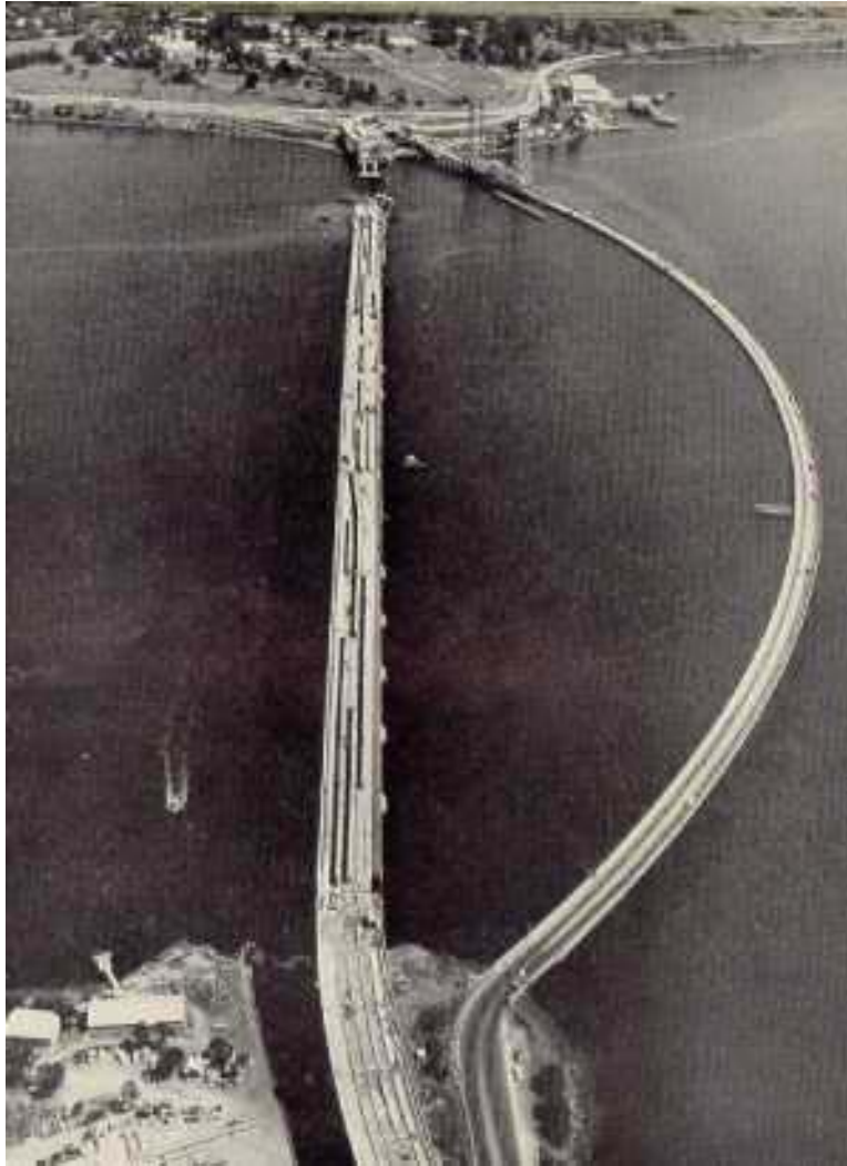
Figure 1.3 – Hobart & Tasman Bridges, Tasmania Photograph obtained from Parliamentary Historical Resources, Parliament of Tasmania http://www.parliament.tas.gov.au/history/hobartbr.htm
