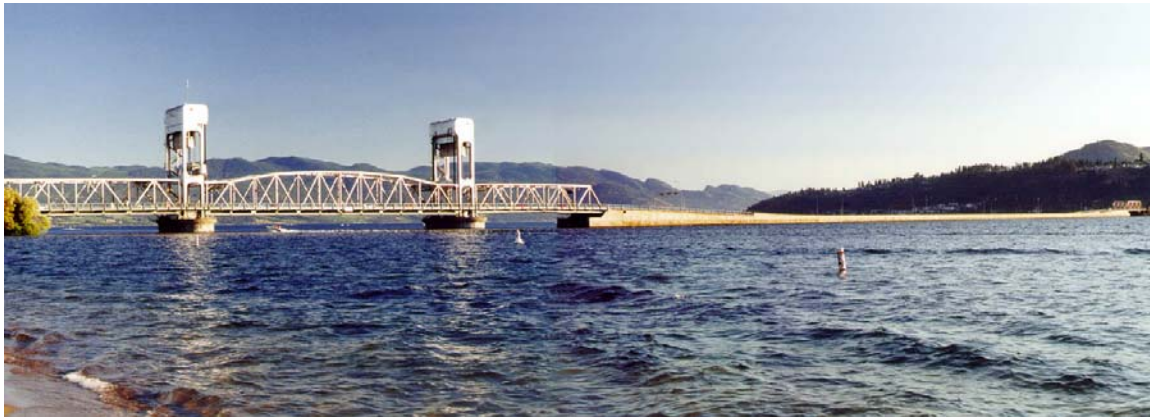
Figure 1.4 – Lake Okanagan Floating Bridge
